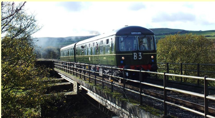
The 105 heading north near Ewood Bridge
